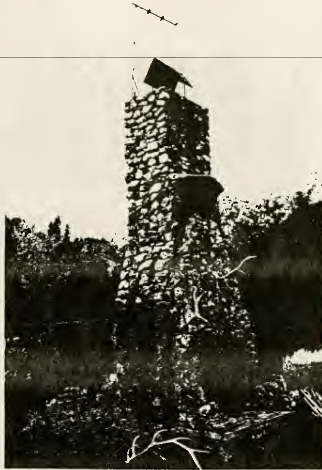
Figure 191. Structure #69, northwest view.
